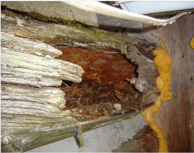
Damaged logs near kitchen on bar wall. Picture taken August 2003.
